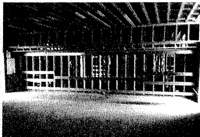
Interior Classroom Framing
